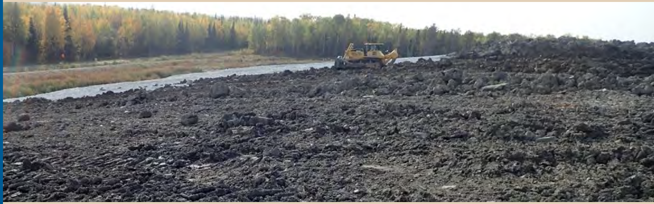
SE Corner of EMRS North of Teeple Road
